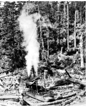
Logging started in Gillies Bay in the early 1900's and, by 1920, the Alberta Logging Company was the largest on the island. A steam donkey dragged logs down a trough formed by laying three logs alongside each other. The sets of three were butted end-to-end creating a skid road more than half a mile long!
